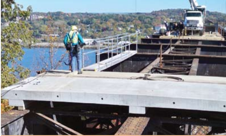
Above: Panels being placed on the bridge. Right: View of the bridge
