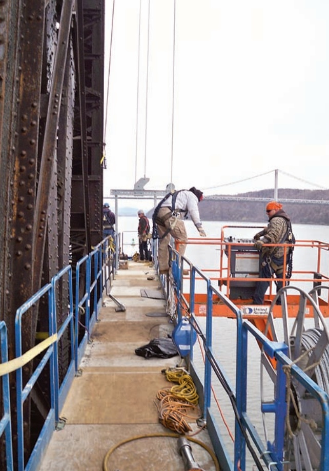
▲ Chill. Work in high winds over the river was a challenge.
