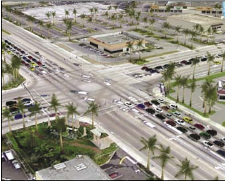
FDOT - Existing Conditions
