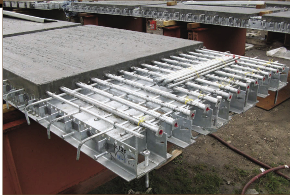
Precast Exodermic Bridge Deck Panel
