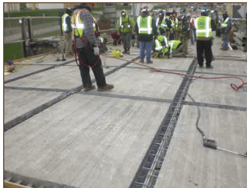
Precast Bridge Deck Panel Ready for Grouting of Closure Pours
