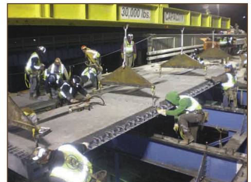
Precast Bridge Deck Panel Being Lowered Into Position
