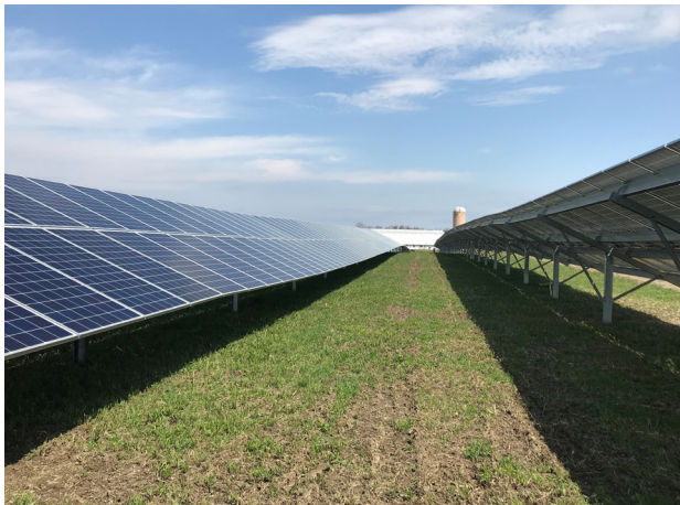
One of the solar power projects Bergmann has worked on. (Provided photo)
