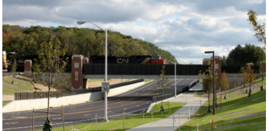
Farm Lane Road & Rail Grade Separation, East Lansing MI
